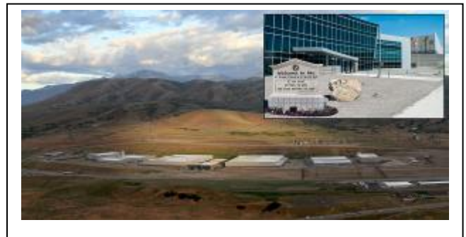
Fig. 1. Utah Data Center [Source: https://nsa.gov1.info/utah-data-center/ ]
